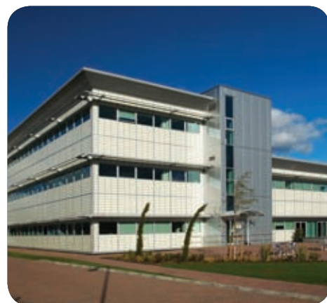
Leicester, UK, HQ for Office Depot ISO 14001 certified
